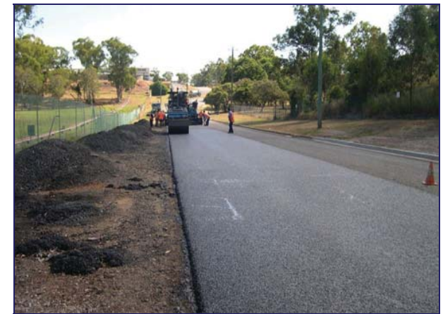
SMA Production and Placement Trials
